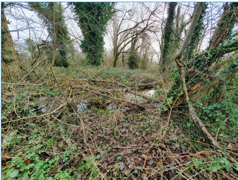
An example of the scrub next to the brook that will be removed to allow plant access for silt removal
